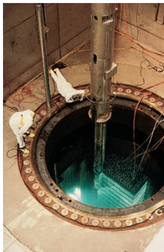
Figure 21.11 Refueling the core of a nuclear reactor.
