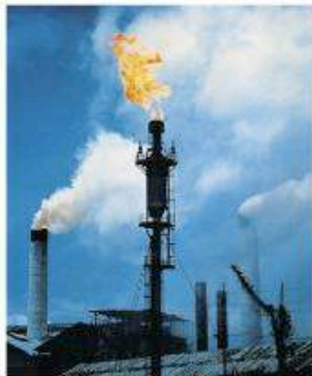
Figure 14.2 The flare stack at an oil refinery is a safety device. If a process goes wrong (for example, if pressures get too high), reactants and products can be sent to the flare stack, where they burn off safely.
