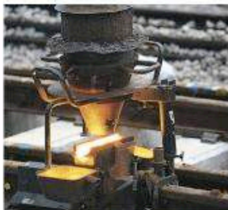
Figure 8.1 Rails are welded together using molten iron, produced by a reactivity series reaction between aluminium and iron(III) oxide.
