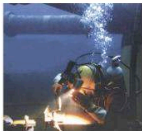
Figure 14.3 The burning of hydrogen is used in oxy-hydrogen cutting equipment underwater.
